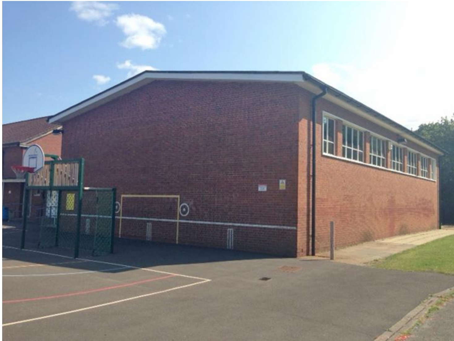
Figure 1 : Existing rear elevation of the school in vicinity of application site
