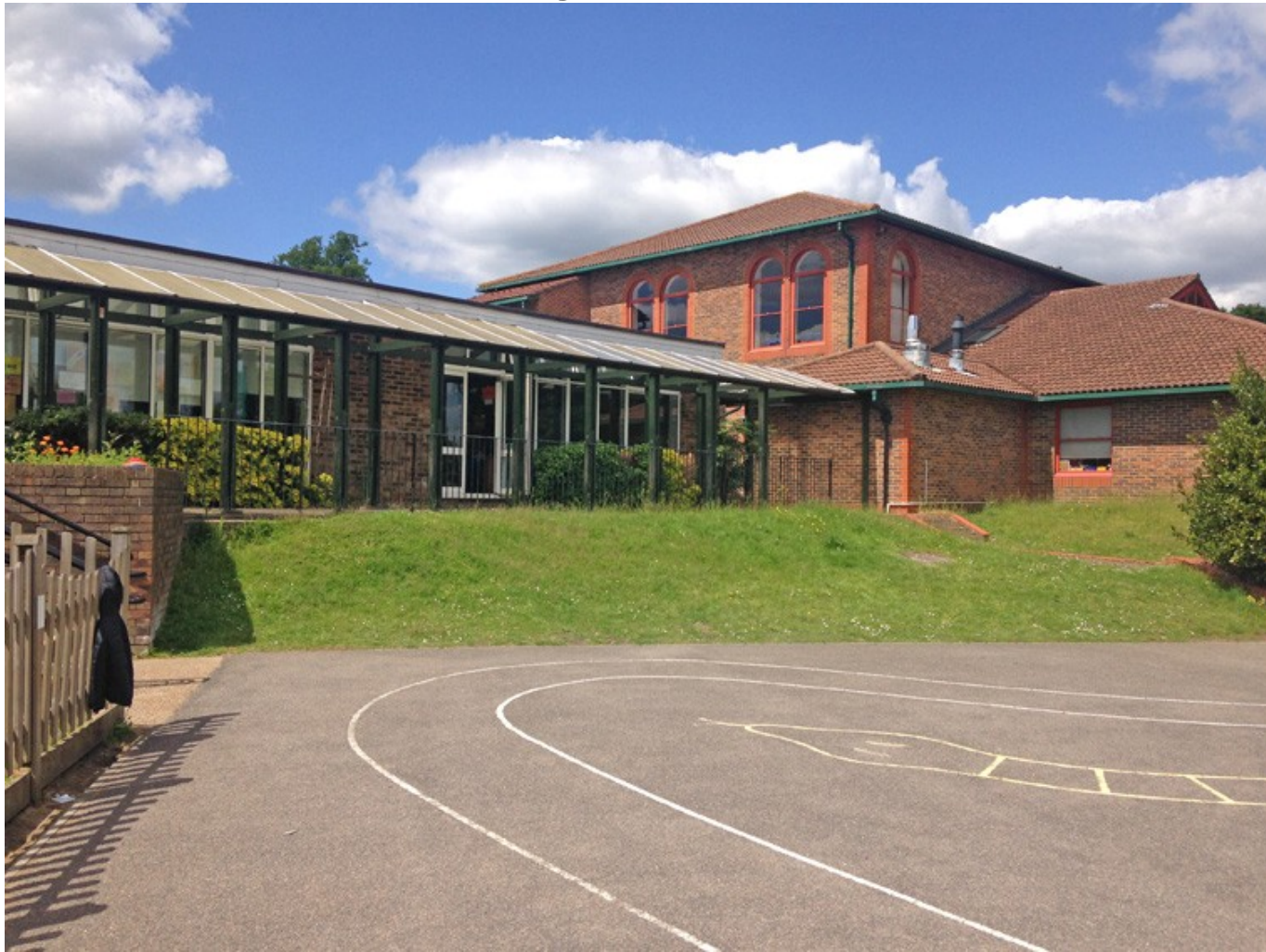
Figure 6 : View of the location of the reception play area alterations and proposed ramped access facing north west
